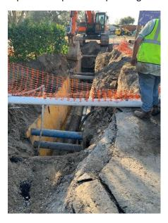
• Gruhn May, Inc. removed the temporary effluent bypass and reinstalled the removed sections of force main to put the effluent line back into service.
