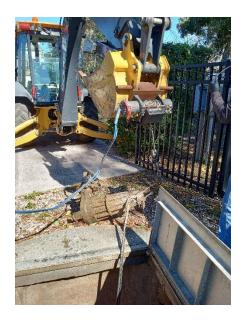
• D&C repaired a water break in the 200 block of Bowles Street.
