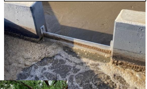
Sluice Gate (adjustable weir) between anaerobic and aerobic basins
