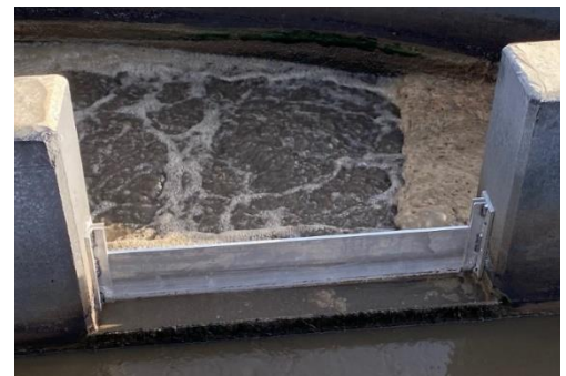
Sluice Gate (adjustable weir) between anaerobic and aerobic basins
