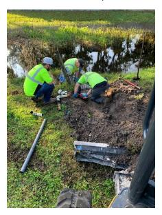
• D&C repaired a sewer lateral at 1321 Penman Road to replace the old VCP with PVC.
