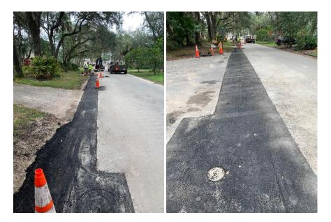
• Stormwater and D&C installed a replacement inlet at 1515 Strand.
