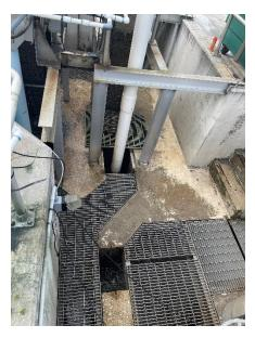
• D&C repaired a water break at 741 Camelia Terrace caused by tree roots.
