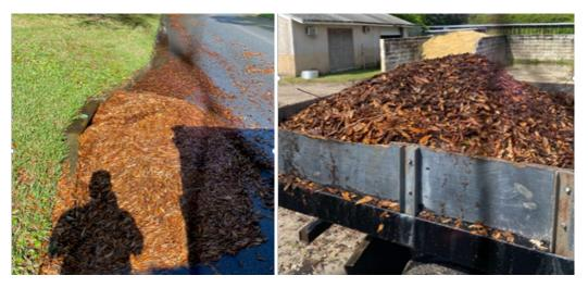
• Stormwater temporarily pulled the gutter protection at 3<sup>rd</sup> and Lemons Street on the FDOT's project so the water would drain out of the travel way in the best interest of the public's safety. We followed up with an email to the FDOT requesting that their Contractor inspect the erosion and sediment BMPs on the project.
