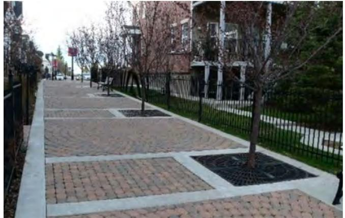
Figure 4.87: Pervious pavers with tree wells
