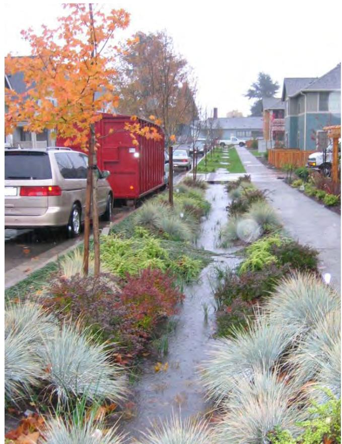
Figure 4.88: Bioswale filters stormwater
