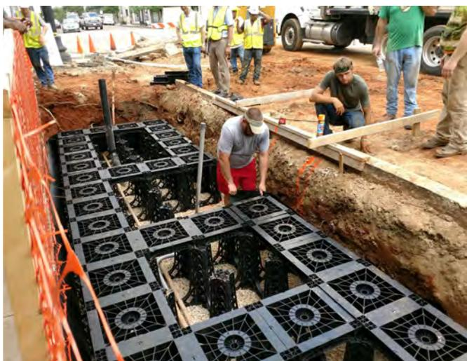
Figure 4.86: Tree wells with Soil Cells
